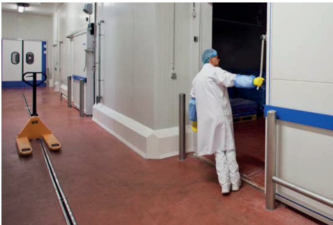
POLYSTO IP40F SANICOAT INSTALLED ON A CONCRETE FLOOR AND STAINLESS STEEL POSTS AND BARRIER BUILT IN A CONCRETE FLOOR.
