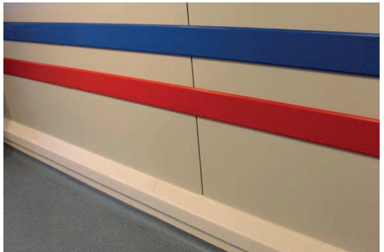
POLYSTO OP30RB (OPTIONAL EXTREME IMPACT) WITH EPOXY FLOOR COVING APPLIED IN TO A REBATE AND RED AND BLUE PE WALL STRIPS.
