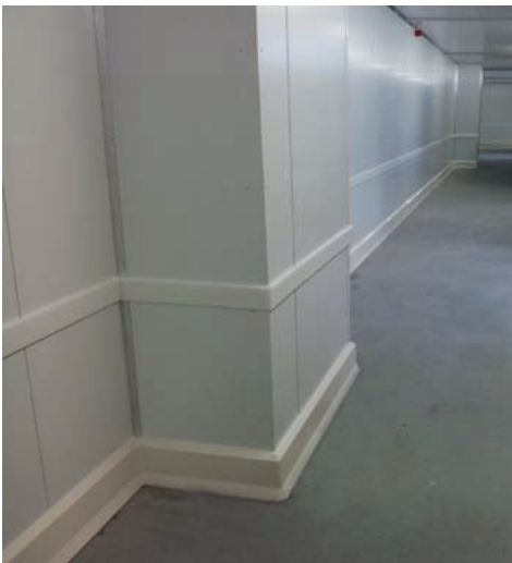
POLYSTO OP20F INSTALLED ON A CONCRETE FLOOR WITH PE STRIP.
