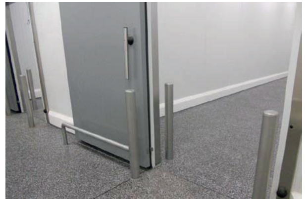
POLYSTO BUILT IN STAINLESS STEEL POSTS AND BARRIER AND OP30RB SANICOAT WITH GRANITE FLOOR COVING APPLIED INTO A REBATE.
