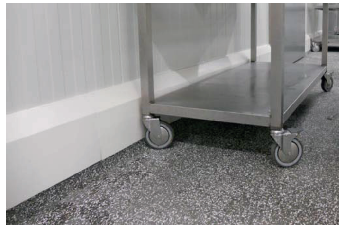
POLYSTO OP30RB WITH GRANITE FLOOR COVING APPLIED INTO A REBATE.
