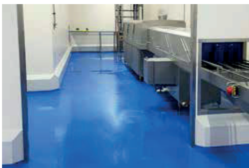
POLYSTO IP40RB NATURAL WITH EPOXY FLOOR COVING APPLIED INTO A REBATE.
